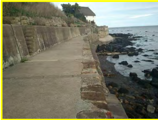
Overview of wall, Oct 2012. (Asset Ref. 1221D901D0601C03)
