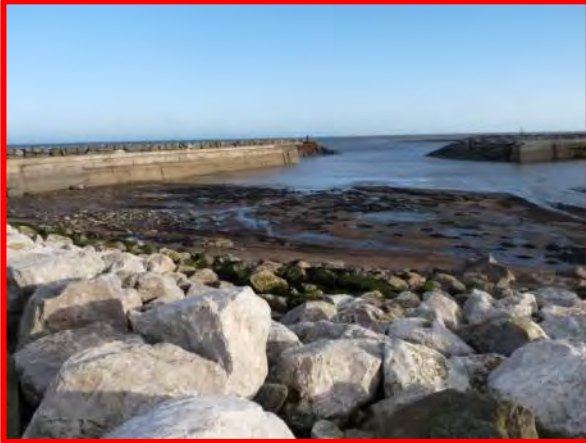
MU4/1a Beach condition after the December 2013 storm surge. (Totally Active)
