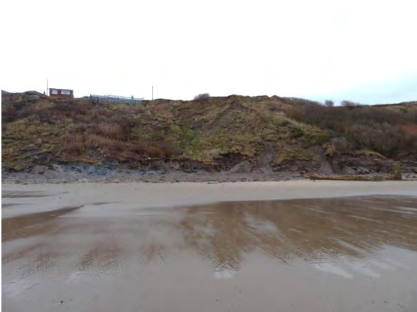
MU29/AQ – December 2013. Substantial toe erosion. (Partly Active)
