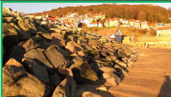
Runswick Bay village rock armour defences, 17 th December 2013. (Asset Ref. 1221D901D0602C01)
