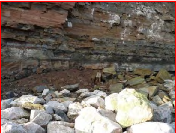
MU4/1a Close up photo of talus accumulation behind rock armour after the December 2013 surge. (Totally Active)
