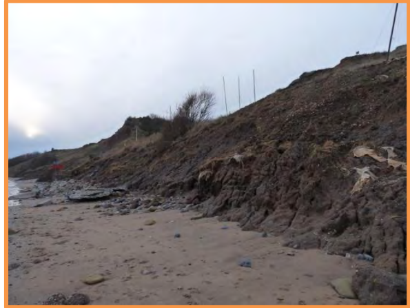
MU27/T – Southern end of unit. Note recent toe erosion throughout unit. December 2013 (Partly Active)
