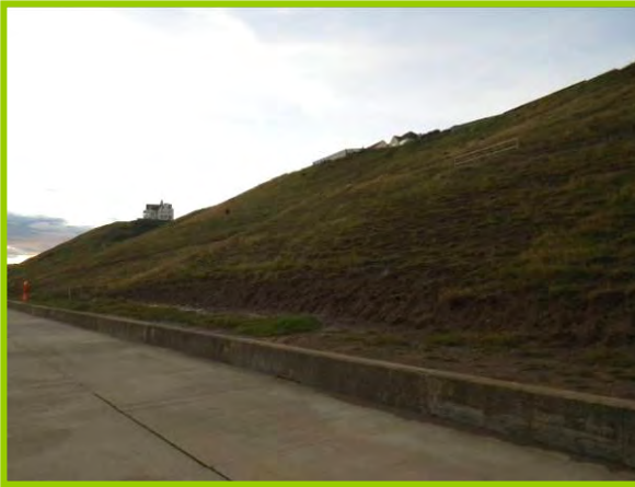
MU11/1 Regraded, stabilised slopes (Inactive) Oct 2012
