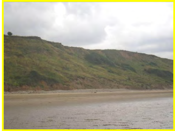
MU29/AF Well vegetated with some toe erosion (Locally Active) Sept 2012
