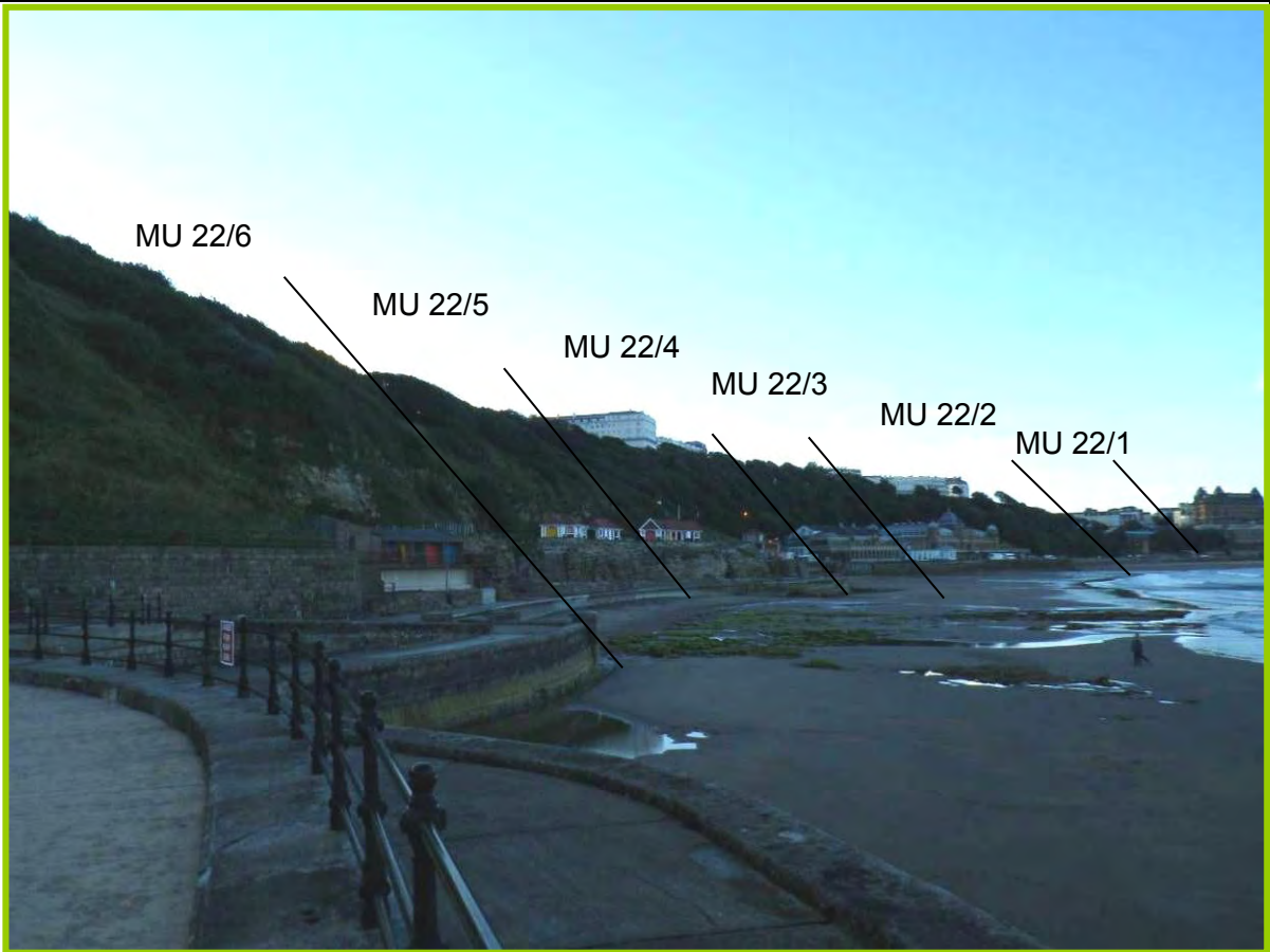
MU22/1 to MU 22/6 Well vegetated slopes with large coastal defences at the toe (Inactive) Sept 2012
