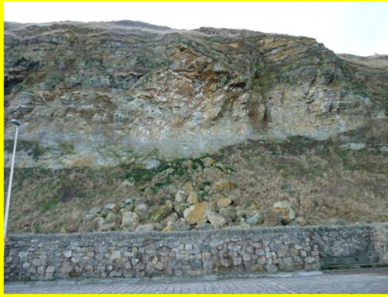
MU21/2 – December 2013. Large rockfall but with significant proportions of the slope still vegetated (Locally Active)
