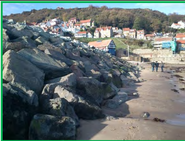
Runswick Bay village rock armour defences, Oct 2012. (Asset Ref. 1221D901D0602C01)
