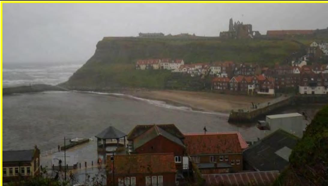
MU12/1 Below Whitby Abbey the slopes are vegetated, but with localised signs of erosion (Locally Active). Cliffs behind Henrietta St (row of white cottages extending along cliff face below St Mary's
