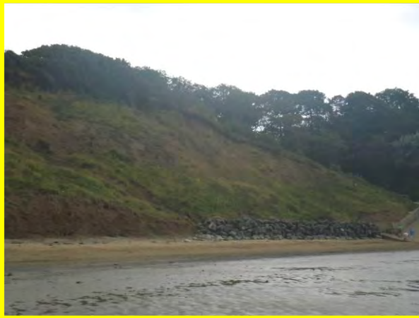
MU29/AA Very common intense erosion and headscarp recession (Locally Active) Sept 2012
