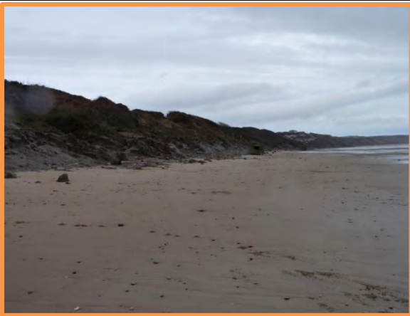
MU29/T – Showing toe erosion and beach condition. December 2013 (Partly Active)
