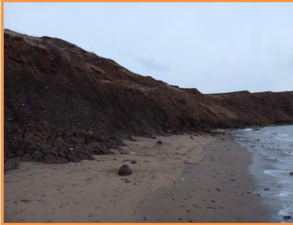
MU27/T – Northern end of unit. Note recent toe erosion throughout unit. December 2013 (Partly Active)
