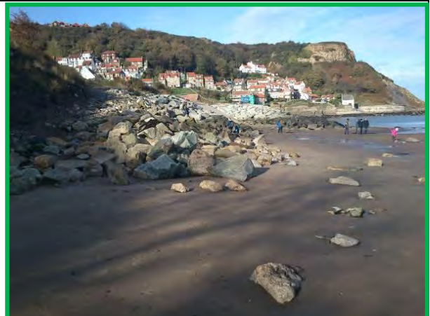
Southern end of Runswick bay rock armour defences, Oct 2012. (Asset Ref. 1221D901D0602C01)
