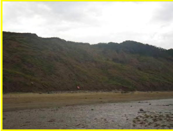
MU29/AB Eroding toe and sliding mid-slope (Locally Active) Sept 2012
