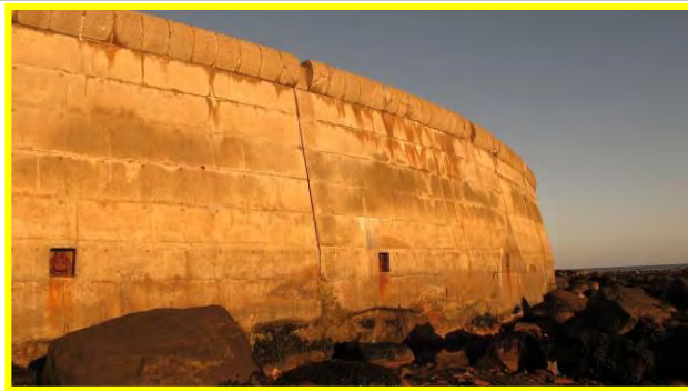
Northern coastal seawall, 17 th December 2013 (Asset Ref. 1221D901D0601C01)
