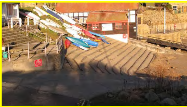
Northern slipway adjacent to the RNLI, 17 th December 2013. Some timbers now missing. (Asset Ref. 1221D901D0601C04)
