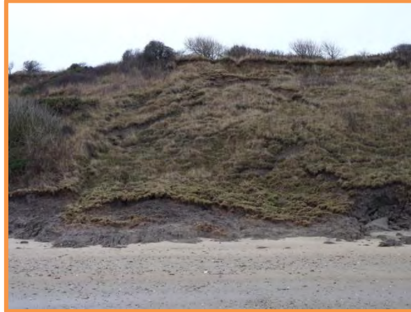
MU29/AH Failure affecting near whole slope. December 2013 (Partly Active)
