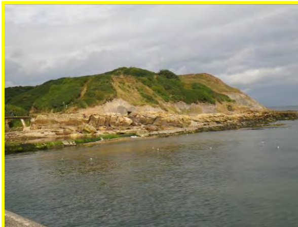
MU19/11 Long Nab is eroding at the toe but the cliff face is well-vegetated and stable (Locally Active) Sept 2012
