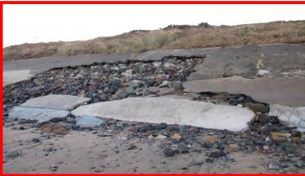
Temporary repairs to revetment voids on 17 th December 2013. (Asset Ref. 1221D901D0702C02)
