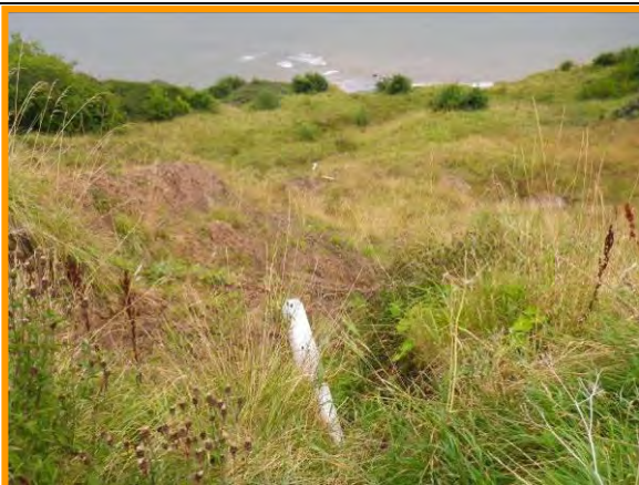
MU17/2 The land drains from the adjacent fields are draining on to the cliff and causing instability (Partly Active). Sept 2012
