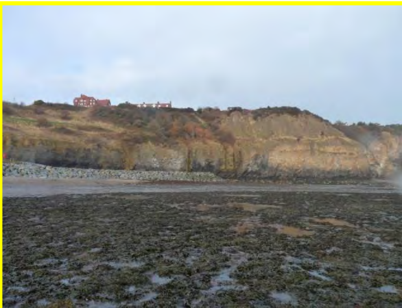
MU16/2 Northern half of MU 16/2, December 2013. Note increase activity beyond end of defences (Locally Active)
