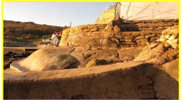
View of northern end of concrete bagwork, 17 th December 2013. (Asset Ref. 1221D901D0601C06)
