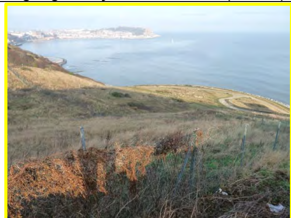
MU22/8 – Locally Active. On the day of survey a small amount of flow was issuing through the rock armour at this toe. 2013
