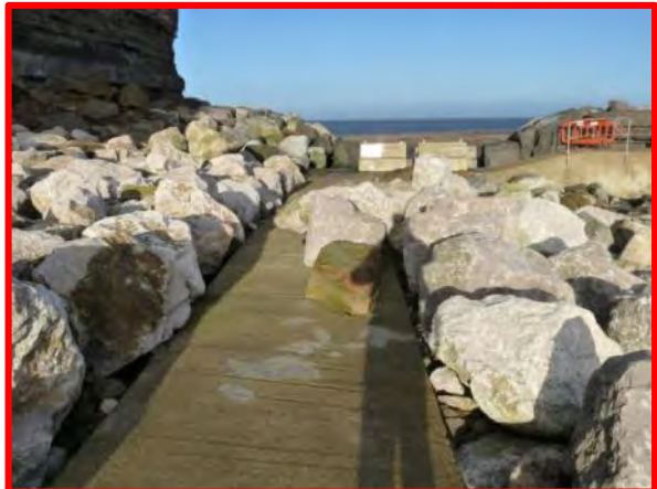
MU4/1a Displaced rock armour and rockfall block on path after the December 2013 surge. (Totally Active)
