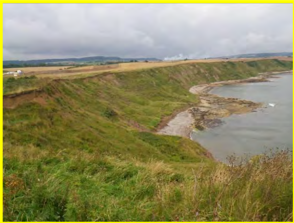
MU19/9 There is evidence of headscarp erosion and erosion of the toe (Locally Active) Sept 2012
