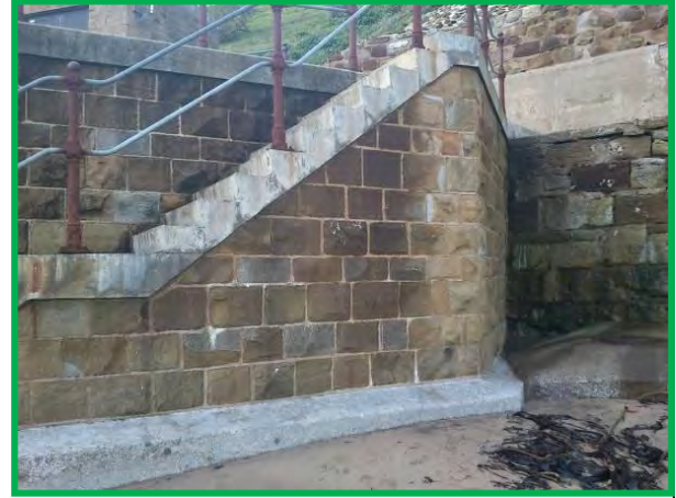
Seawall around the pumping station, Oct 2012. (Asset Ref. 1221D901D0601C07)
