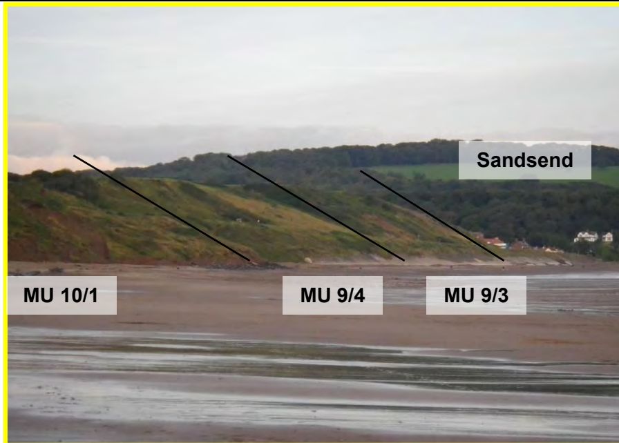
MU9/3 and MU 9/4 The slope overall is stable with erosion apparent at the shore where the defence has become degraded (Locally Active). October 2012
