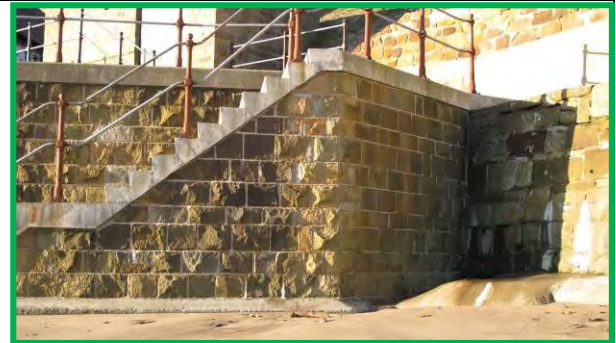
Seawall around the pumping station, 17 th December 2013. (Asset Ref. 1221D901D0601C07)
