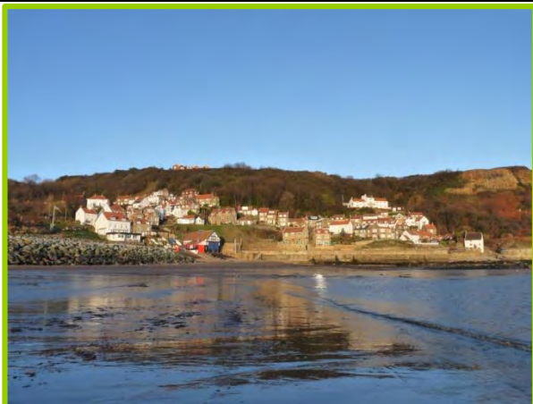
MU7/1 – Runswick Bay Village post December 2013 Storm Surge. Inactive
