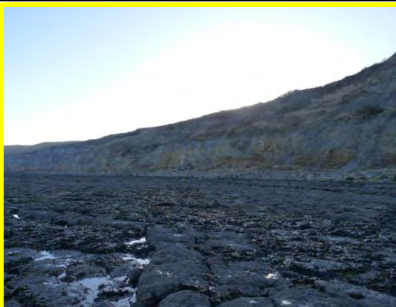
MU23/C - December 2013. Toe erosion throughout (Locally Active).
