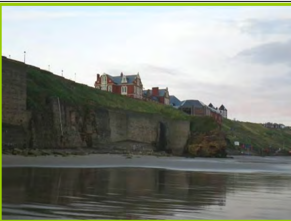
MU11/3 Defended slopes with little evidence of recent activity (Inactive)
