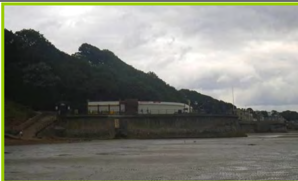
MU28/Y and Z The Filey frontage does not show any signs of slope failure (Inactive). Sept 2012
