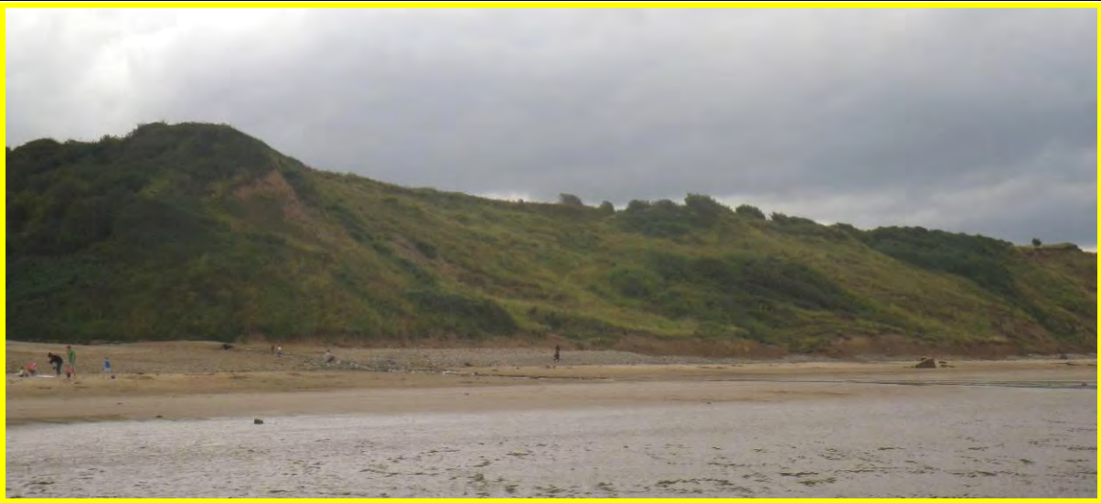
MU29/AI Locally steep, exposed unit toe (Locally Active) Sept 2012
