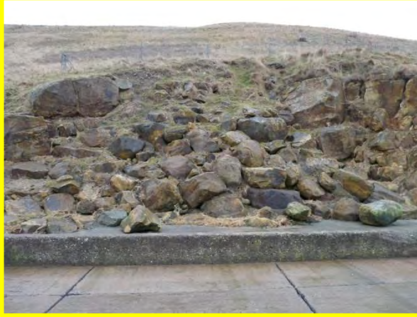
MU11/1 – Recently chipped and moved rockfall blocks at eastern end of unit. December 2013. (Locally Active)
