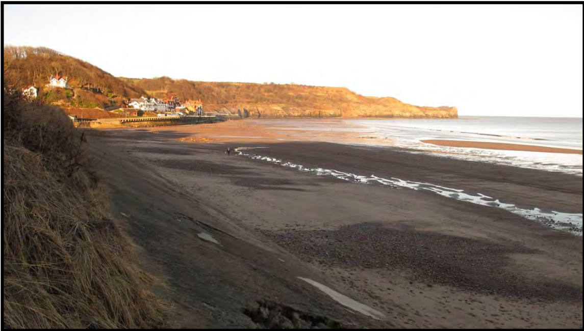
General view of Sandsend beach looking North West with beach levels on 17 th December 2013. (Asset Ref. 1221D901D0702C02)
