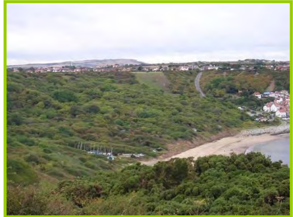
MU7/2 (right of image with rock armour at toe - Inactive) MU7/3 (left with eroding toe – Locally Active). September 2012
