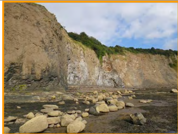
MU16/1 the base of the cliff continues to erode. The undercutting of the cliff is evident in the left side of the photograph (Partly Active) Sept 2012
