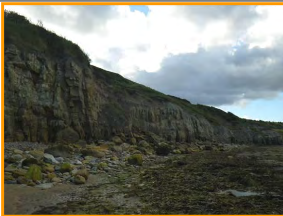
MU23/A Erosion of the toe (Partly Active) Sept 2012
