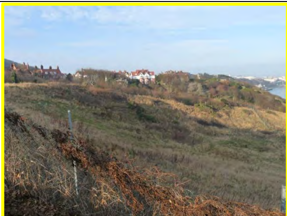
MU22/8 – Locally active (note small slips in scarp). December 2013 (Locally Active).
