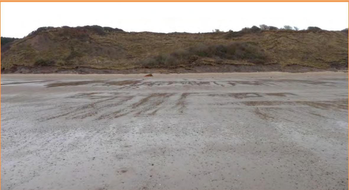
MU29/AI - Whole unit, December 2013. Continues to have locally steep exposed toe throughout unit. Erosion here possibly less severe relative to units further north.
