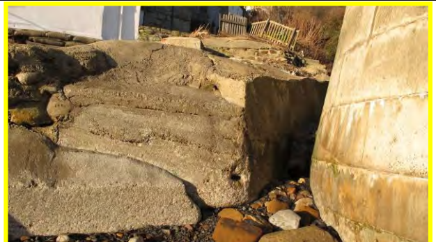
View of Runswick Beck outfall, 17 th December 2013. (Asset Ref. 1221D901D0601C06)
