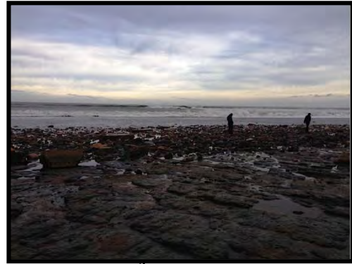
Foreshore on 8 th December 2013, NYCC inspection. (Asset Ref. 1221D901D0702C02)
